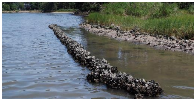
Figure 19 – Oyster reef breakwater (Source: Chesapeake Bay Foundation, 2023)
