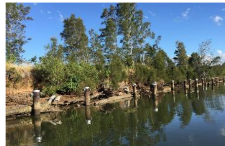
Figures 15 & 16 – Log jam/debris (Source: City of Gold Coast, 2022)
