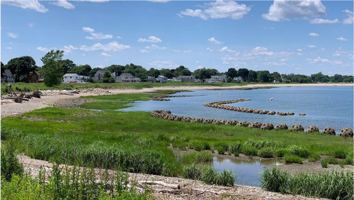
Figure 17 - Reef ball breakwater (Source: Sacred Heart University, 2019)
