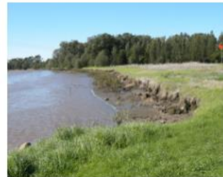
Ash Island (Hunter River NSW) eroding bank before, during and 3 years after installation of rock fillet, showing mangrove seedling colonisation of still water between rock fillet and previously eroding bank
