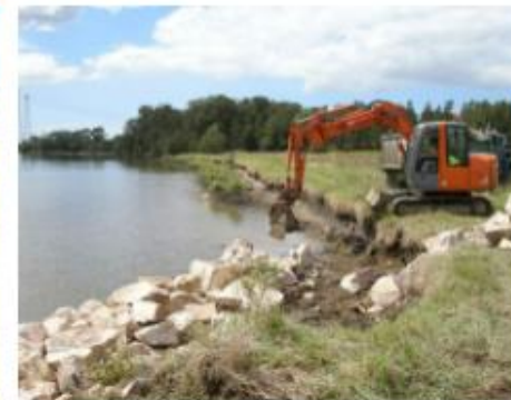
Ash Island (Hunter River NSW) eroding bank before, during and 3 years after installation of rock fillet, showing mangrove seedling colonisation of still water between rock fillet and previously eroding bank
