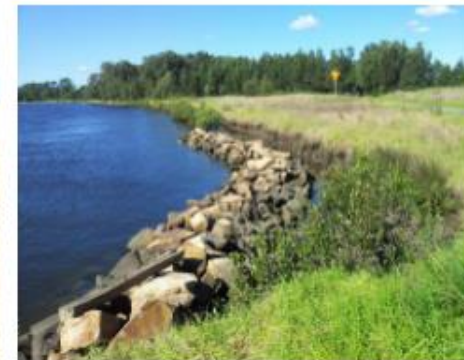
Ash Island (Hunter River NSW) eroding bank before, during and 3 years after installation of rock fillet, showing mangrove seedling colonisation of still water between rock fillet and previously eroding bank
