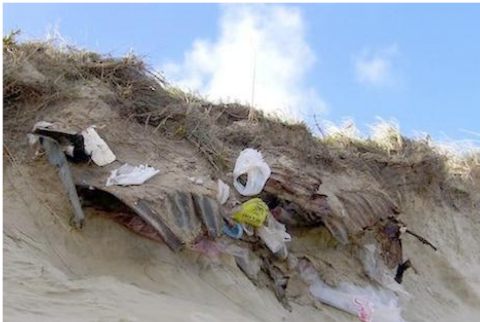
Figure B-7 Port Fairy landfill erosion (ABC News, 2019)
